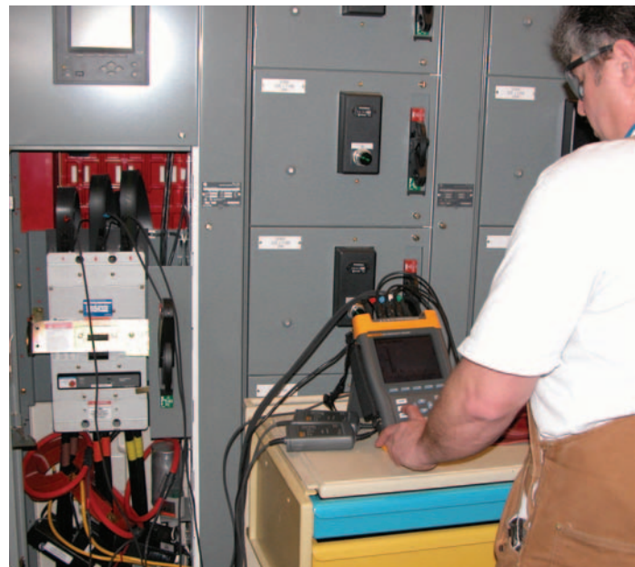
Maintenance Electrical Specialist Mark Newport using a Fluke 434 Power Quality Analyzer to measure, trend, and document the power factor and harmonics correction provided by the plant's new power correction system.
