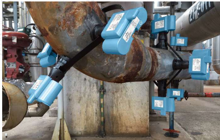
Figure 14: Rosemount Wireless Permasense Corrosion and Erosion Monitoring Systems provide a continuous wall thickness measurement, with data sent via WirelessHART .
