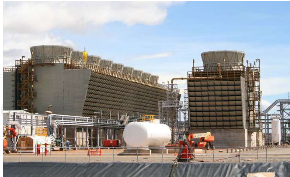
Figure 8: Cooling towers need monitoring because they have complex and often troublesome blower systems, in addition to fluid handling equipment.
